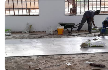
Tiling the Floor of the School
