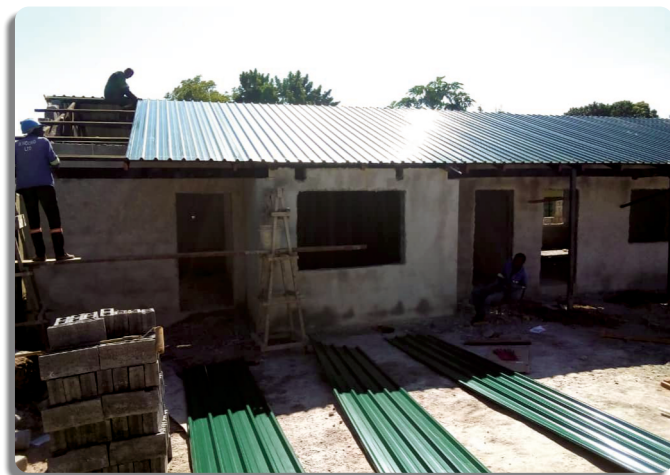
Roofing the New Building
