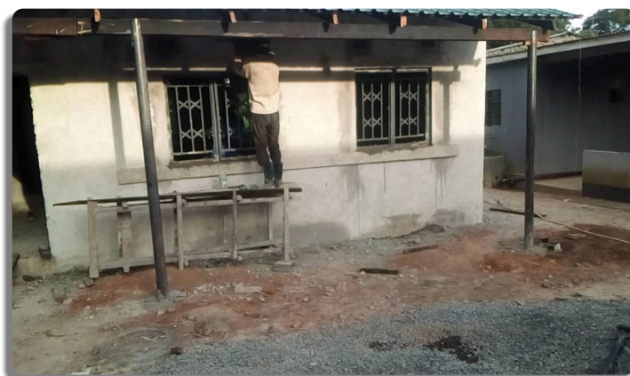
Plastering the Walls
