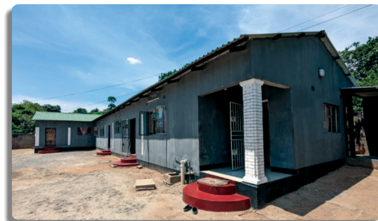
Outside of the Original Building
